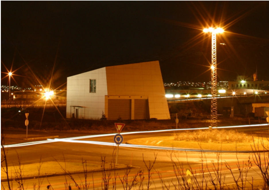
Figure 3: Breivika WWTP in Tromsø
