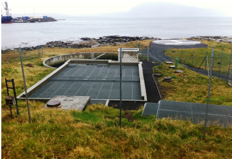
Figure 6: The LSH Main Hospital WWTP in April 2013
