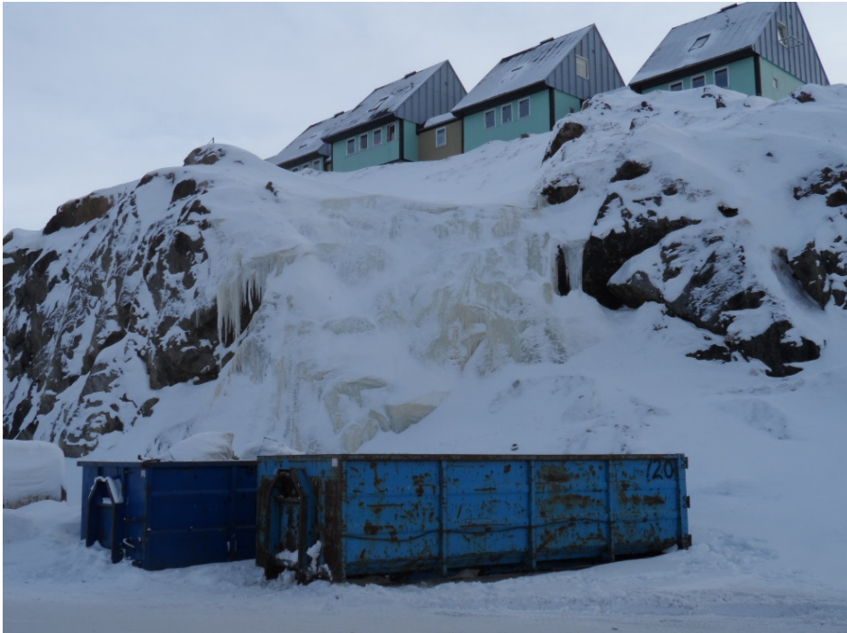
Figure 74: An estimated approx. 15% of total grey wastewater Sisimiut is discharged to terrain
