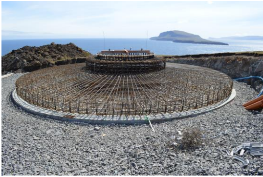
Mynd 3 – Fundament klárt at stoypa
