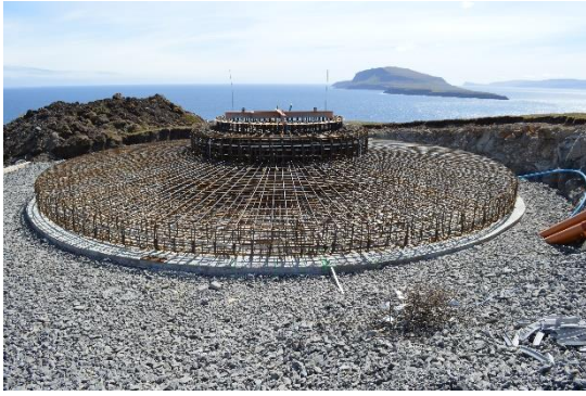
Mynd 3 – Fundament klárt at stoypa
