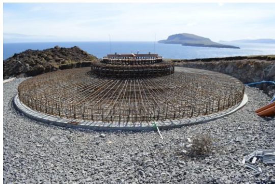
Mynd 10 Fundament, klárt at stoypa
