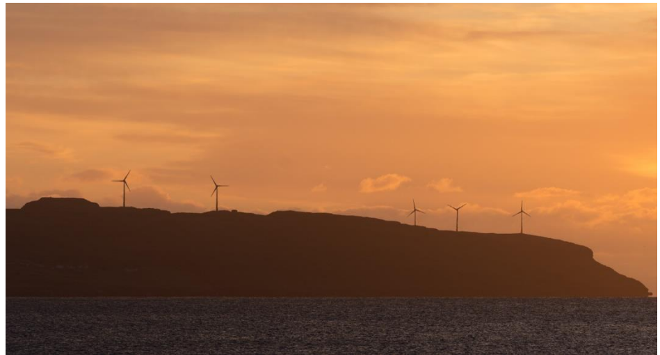
Figure 10: Nesahagi wind farm
